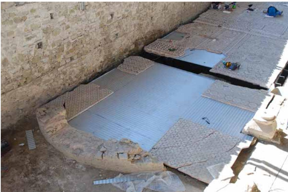
Fig.10 Covering the areas with ribbed aluminum sheets (photo: M. Tutkovski)
