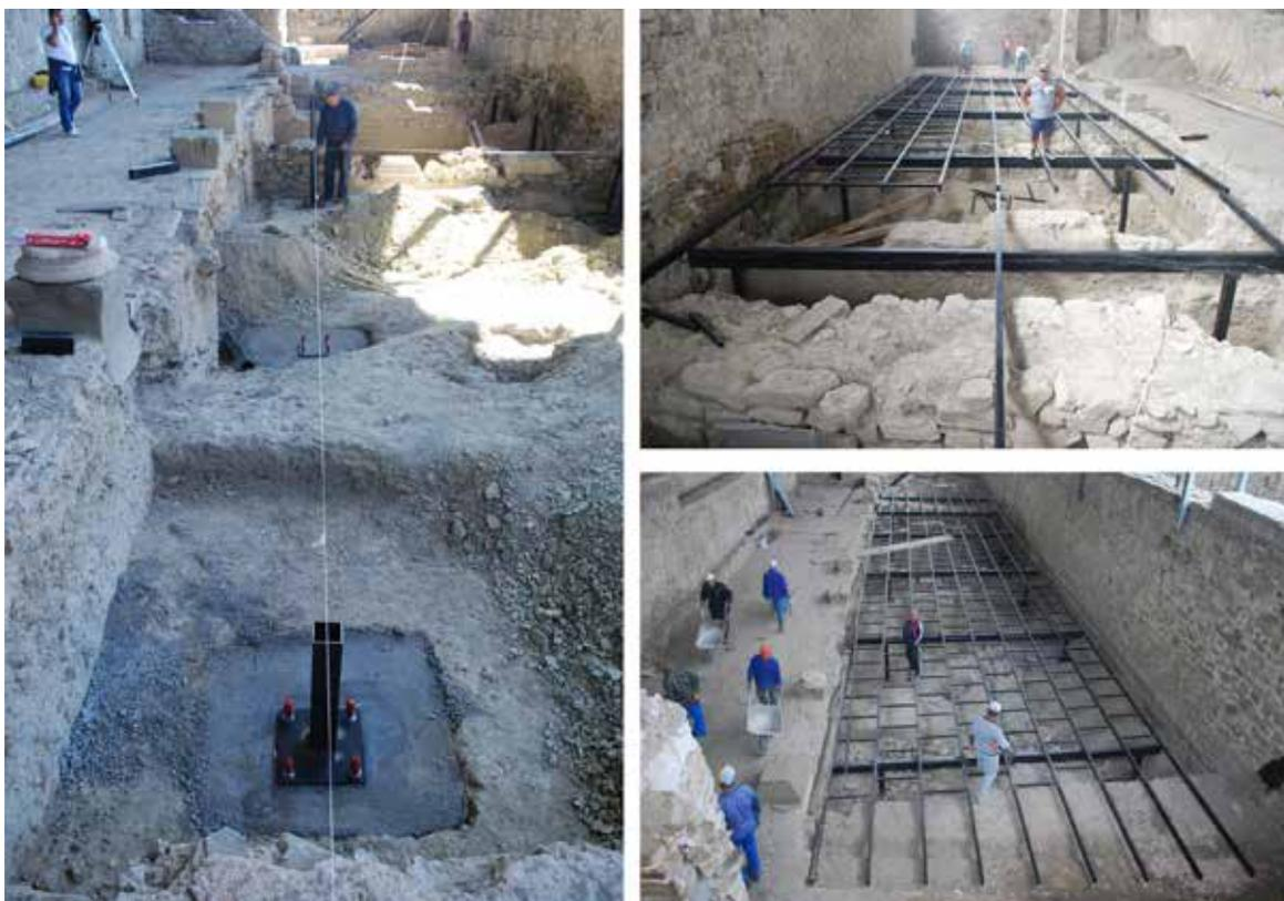
Fig.6 Constructing the steel platform (photo: M. Tutkovski)
